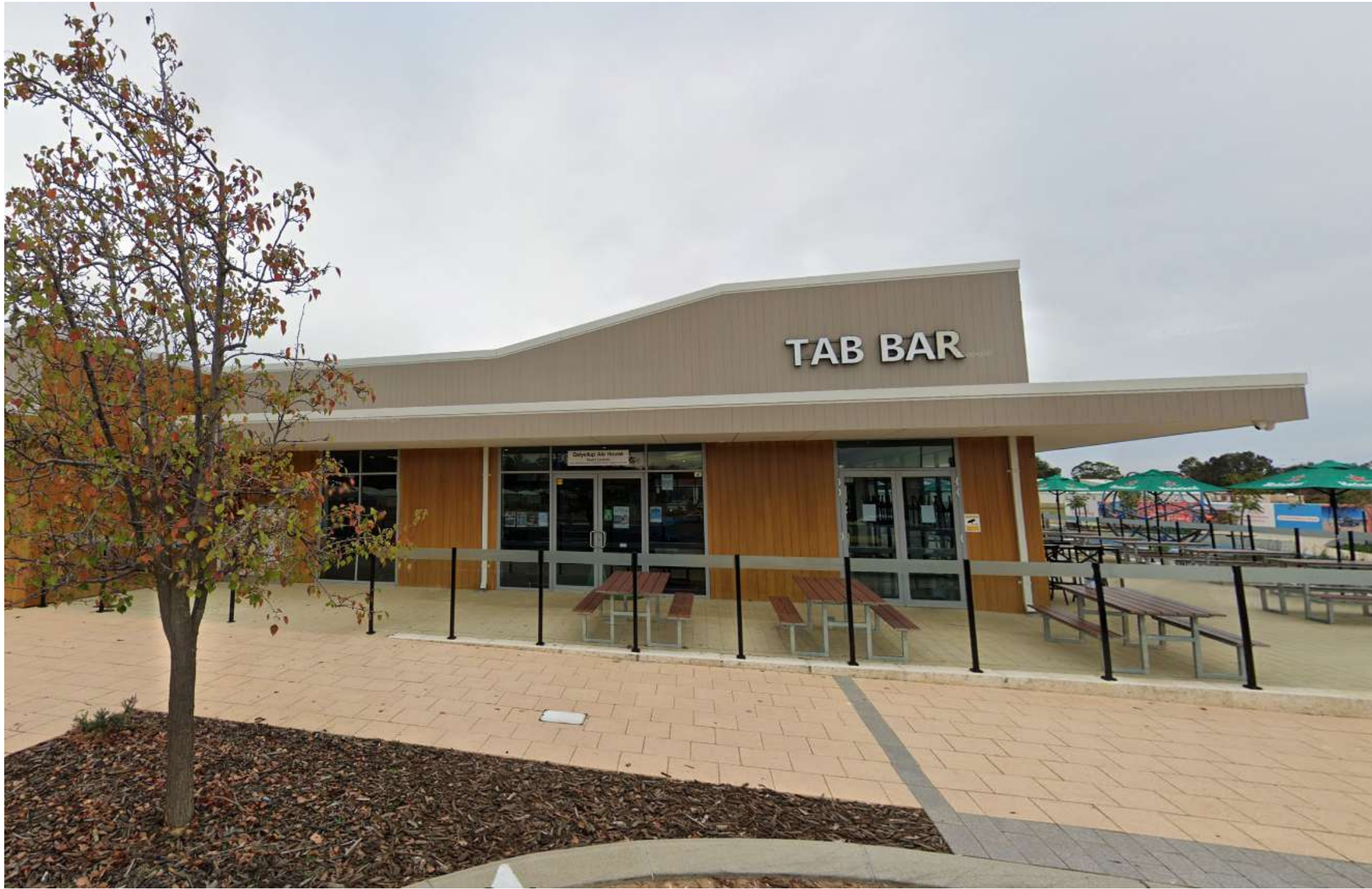
PHOTO TAKEN AT 2 - VERTICAL CLADDING
