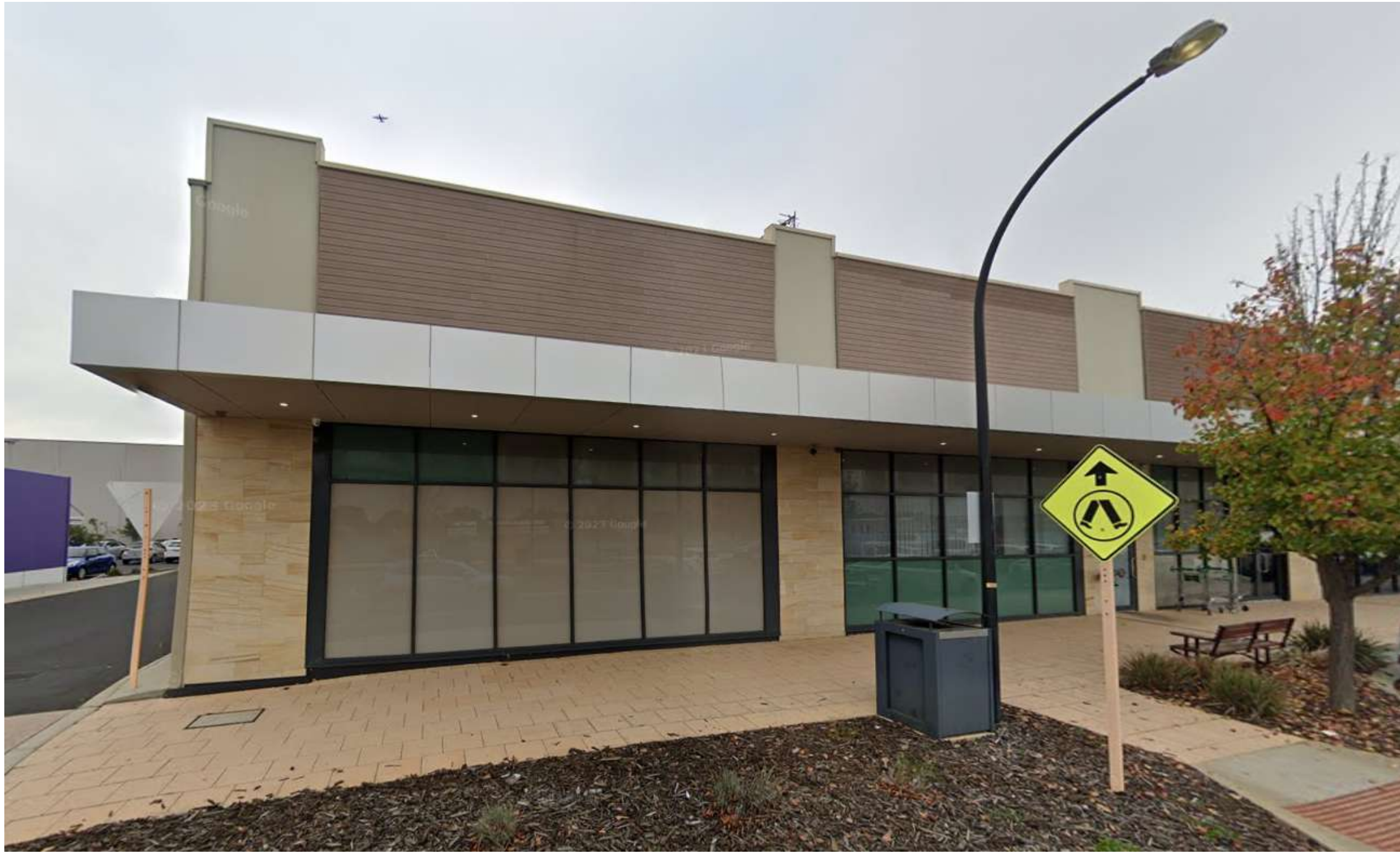
PHOTO TAKEN AT 5 - LIMESTONE LOOK CLADDING
