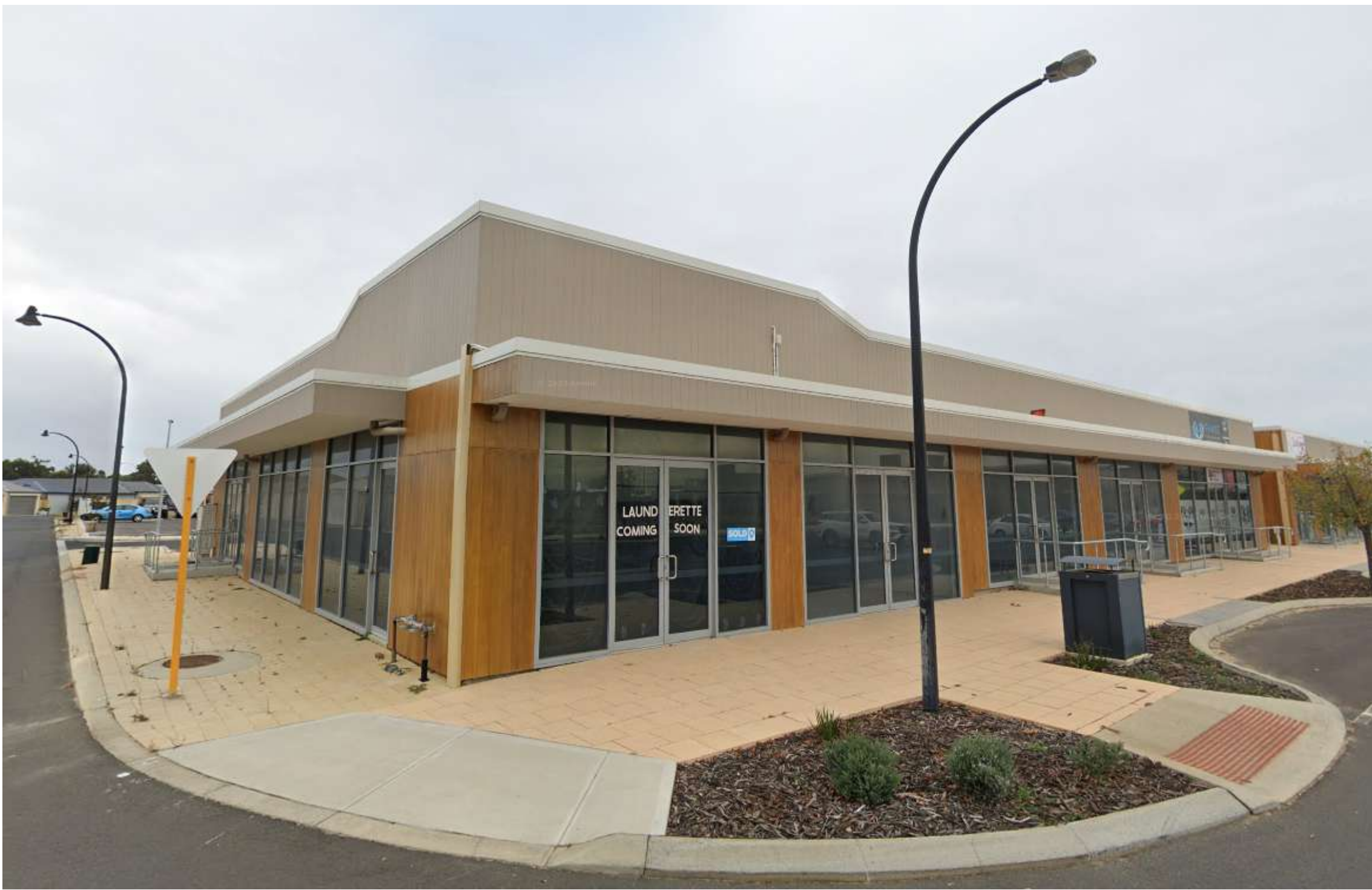
PHOTO TAKEN AT 1 - VERTICAL CLADDING
