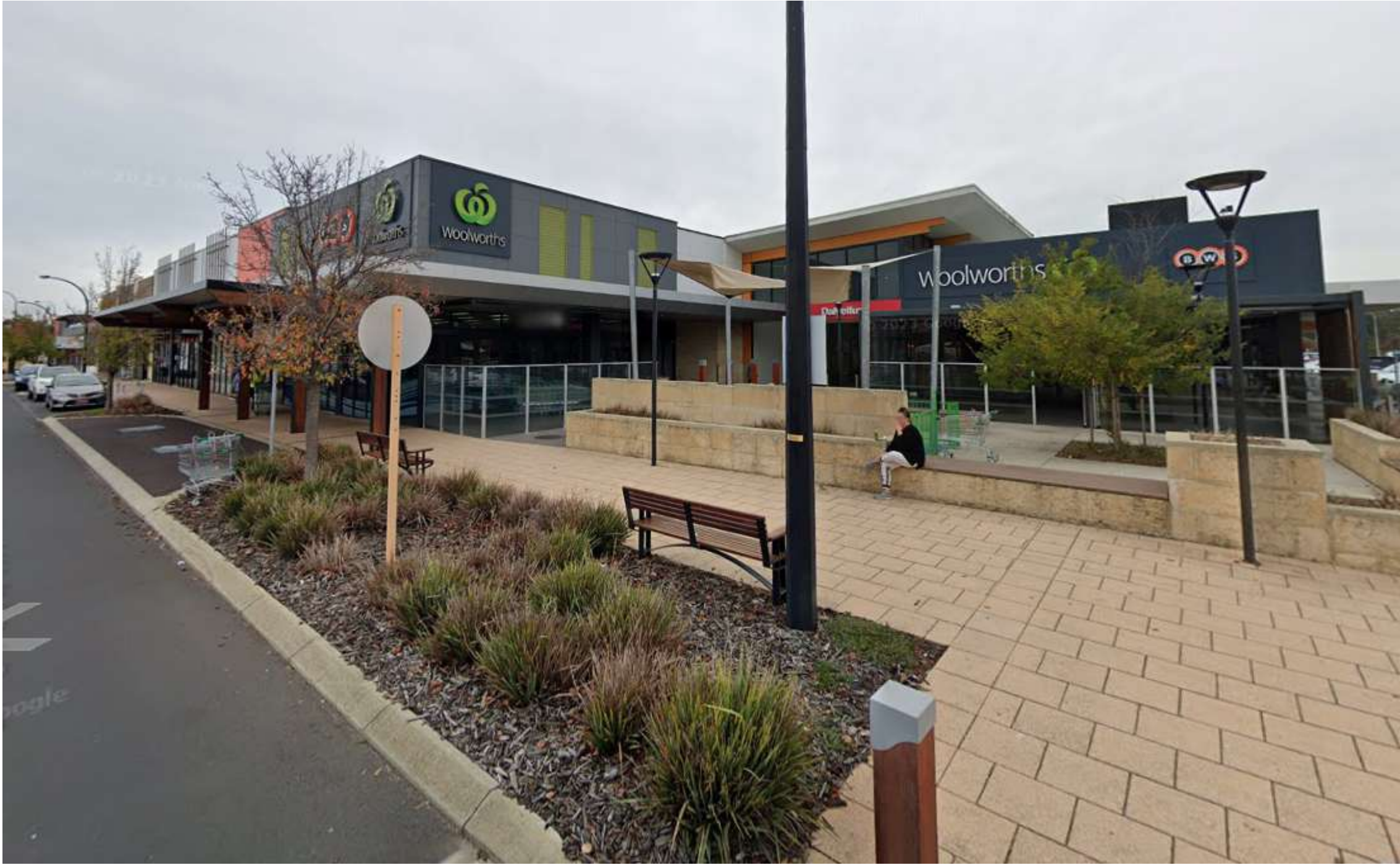
PHOTO TAKEN AT 4 - LANDSCAPE & HARDSCAPE TO ENTRY
