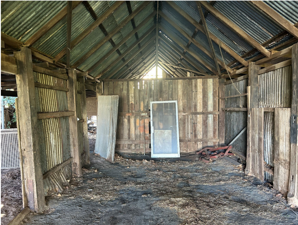
Photograph 21: Internal view of stables building showing poor condition of timber members. Courtesy Doepel Marsh, August 2025.
