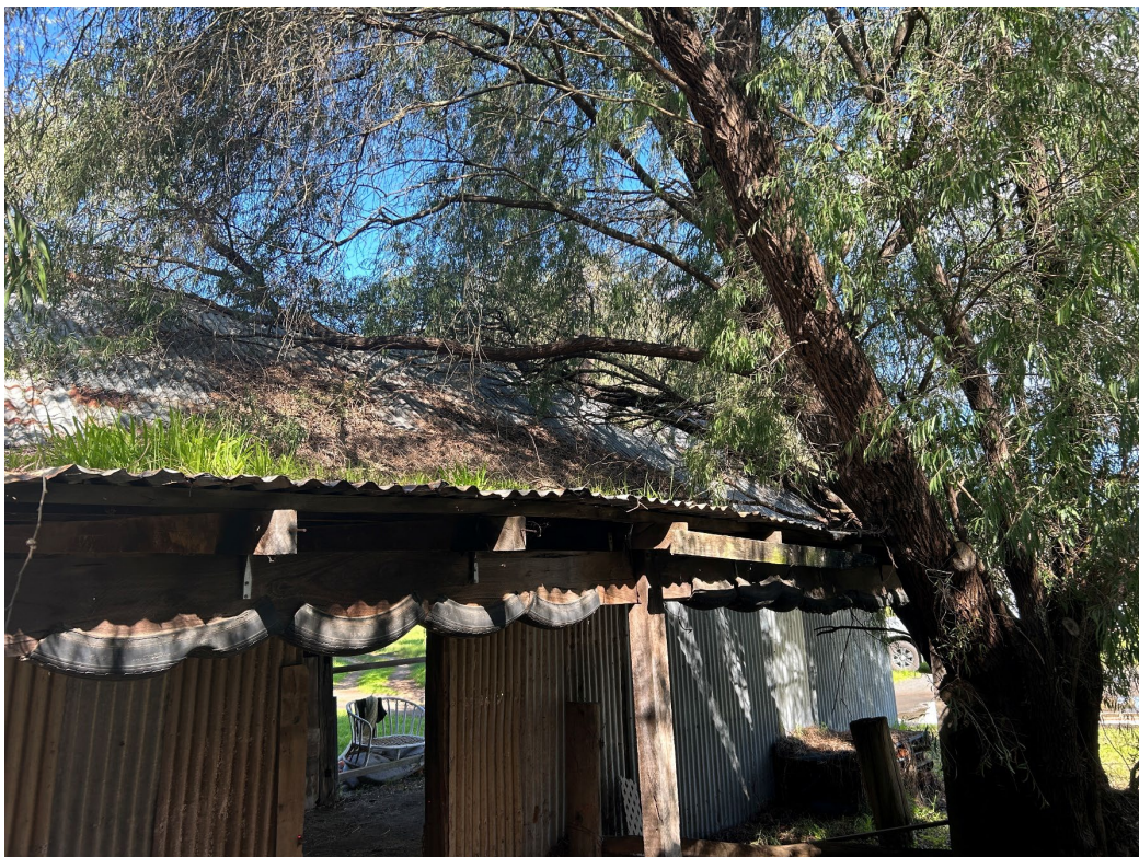
Photograph 16: Damage and other organic growth visible to stable roof structure. Courtesy Doepel Marsh, August 2025.
