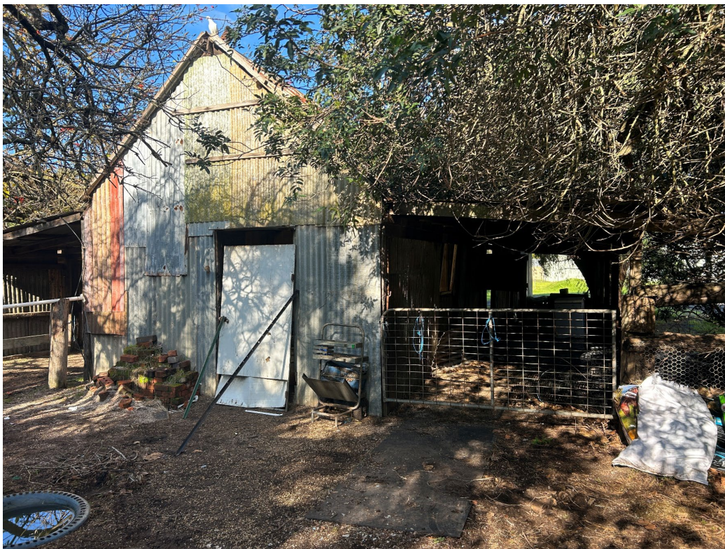
Photograph 18: Looking south-west showing east elevation of stables building. Damage being caused by vegetation and other deterioration visible. Courtesy Doepel Marsh, August 2025.
