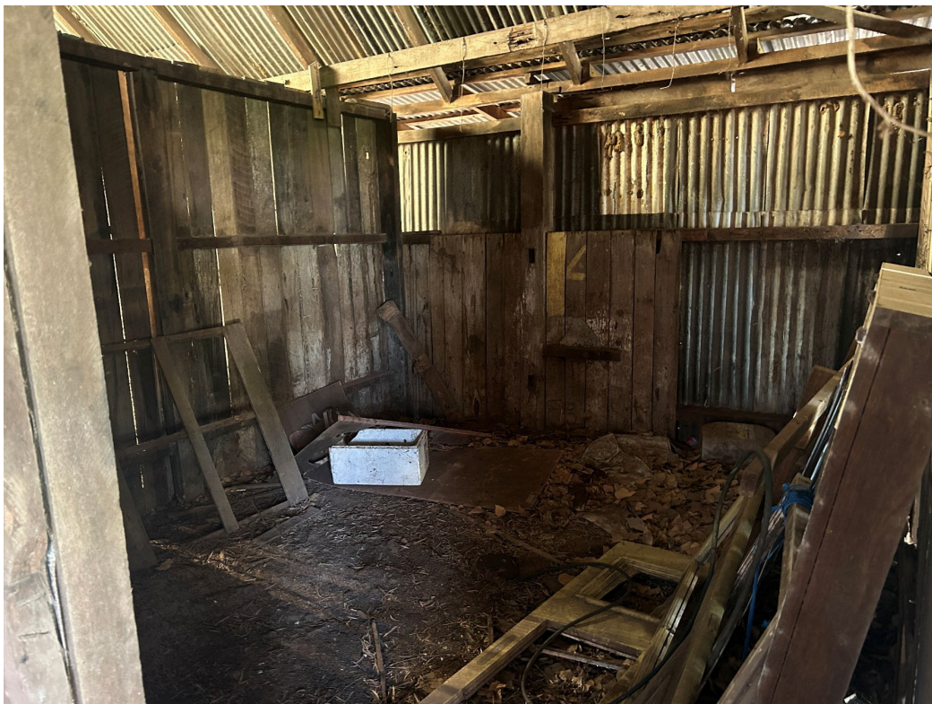
Photograph 20: Internal view of stables building showing poor condition of timber members. Courtesy Doepel Marsh, August 2025.
