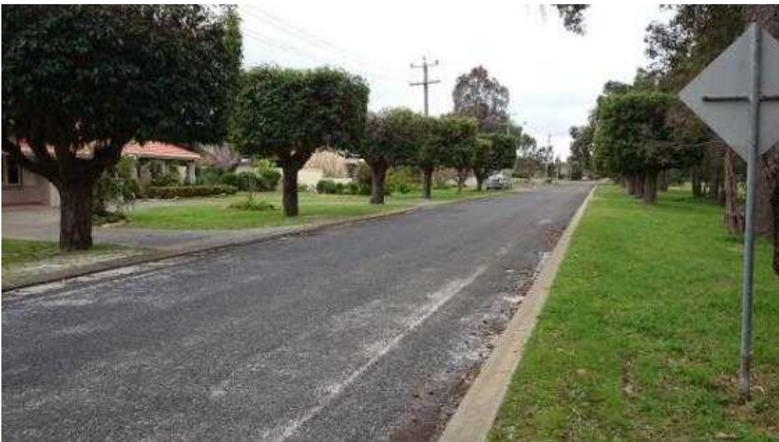
Photo 4: Turner Street, looking east.
