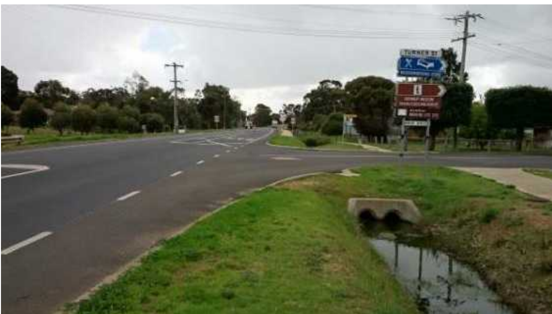
Photo 2: Turner Street intersection looking north along South Western Highway
