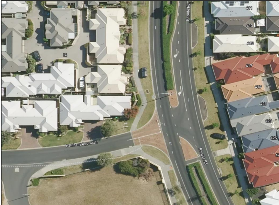
Figure 2-4 Kambany Approach / Parade Road Intersection
