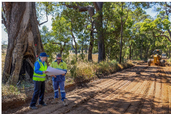
Weld Road widening and gravel re-sheet
