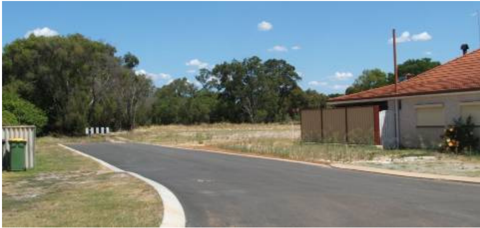
Figure 3 – Starting section of Harrison Road connecting to Roe Road in Precinct 6B
