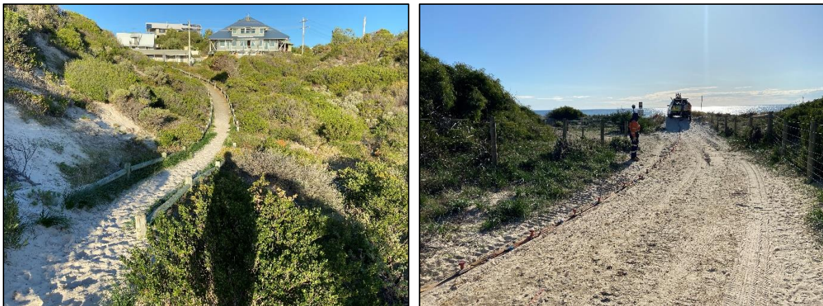
Figure 4: Site conditions at Peppermint Grove Beach including the pedestrian beach access path (left image) and vehicle beach access path (right image).
