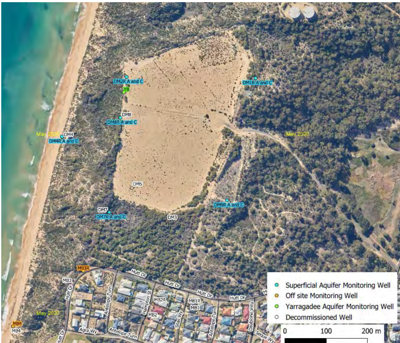
Figure 3 - Monitoring Bore Locations
